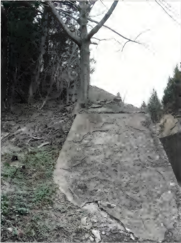
Figure 5.75. View looking southeast at concrete glacis, the Mortar Battery. Here, a tree greater than four-inches in diameter is seen growing directly upon the concrete battery surfaces. Such vegetation must be removed in the interest of long-term preservation of the battery structures (Olmsted Center, April 2008).
